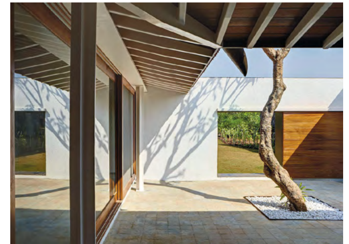
ABOVE Three Court House, Alibag, India, 2014.
